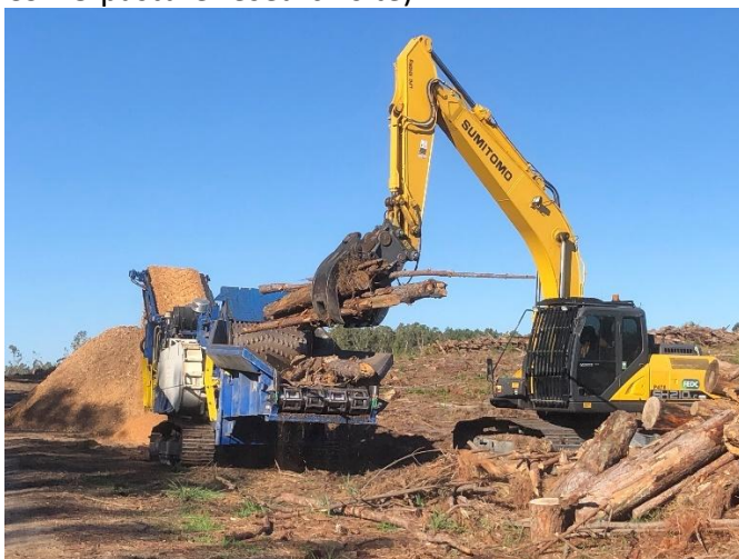
Horizontal flatbed grinder processing roadside stacked CTL harvest debris at Beerburrum before re-loading and transport to a bioenergy facility in northern NSW
